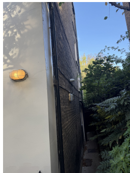
Passage: walls, pipes and foliage
