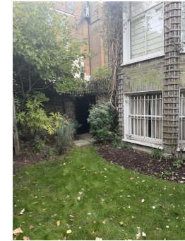
Rear-wing approach and gate area
