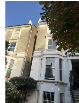
Full front elevation and storeys
